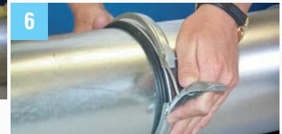
Snap QF Clamp over O-ring and one end of Quick-Fit Sleeve.
